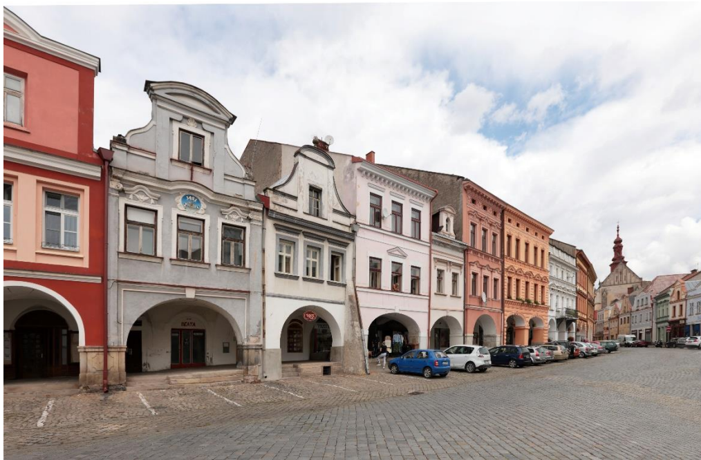
Fig. 19 Jaroměř, Československé armády Square (view from the east), a group of burgher houses with Gothic foundations, arcades and Baroque façades, Gothic Church of St. Nicholas in the background; Zdeněk Rerych 2021
